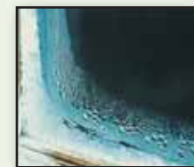
Window condensation fuels mold growth.
