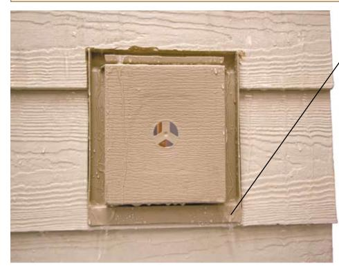
Moisture is the greatest threat to the long-term performance of a home. It can damage the building materials and can lead to an unhealthy living environment. These new blocks help to eliminate the retention of moisture in the exterior home.
